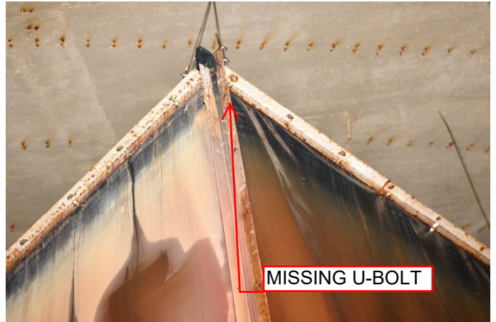
VIEWS OF TYPICAL CORNER CONNECTIONS
