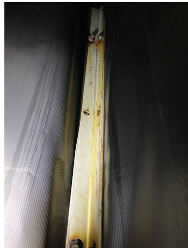
VIEWS OF TYPICAL VERTICAL CONNECTIONS
