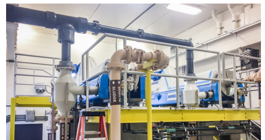
The centrifuges do not need to be constantly watched, there is no water spray and odors are substantially reduced
