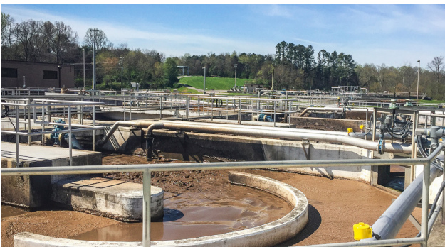
By increasing the volume of sludge in the aerobic digester and adding digester capacity, the detention time for volatile solids destruction increased
