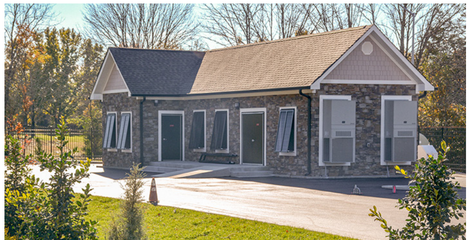
The Windstone Pumping Station was designed to resemble a craftsman style home in order to blend in with the properties in the surrounding area.
